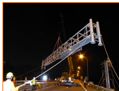
Gantry Erection
