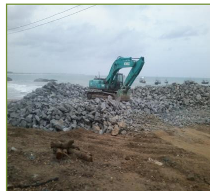
Stock piling of core material at Kalametiya
