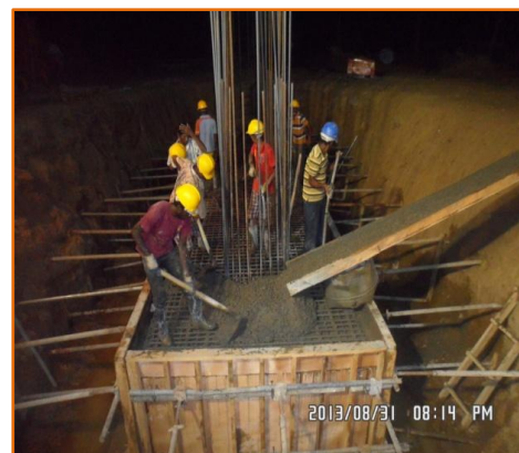
Pier concreting work
