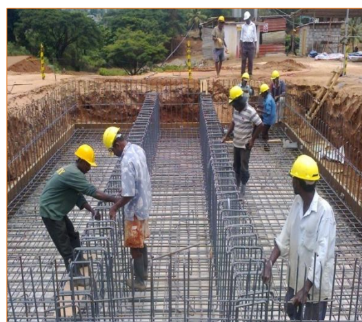
Pallekelle Main Transformer Foundation
