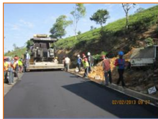
Asphalt concrete wearing course paving
