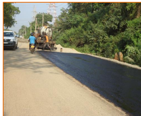
Galkulama - Anuradhapura Road Priming work is in progress
