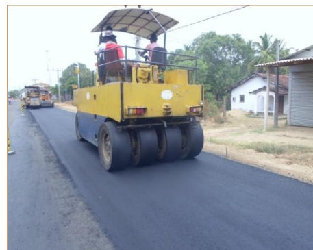
Asphalt concrete wearing course
