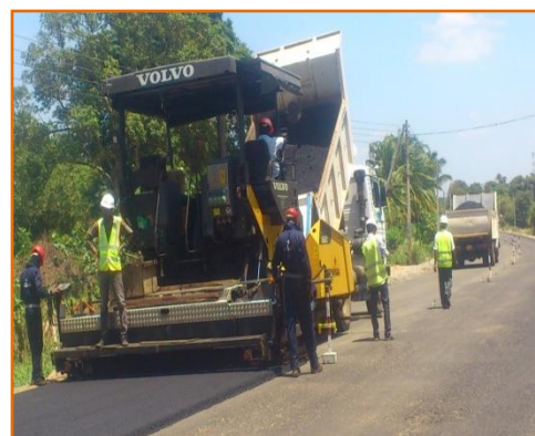
Asphalt Binder Course Laying
