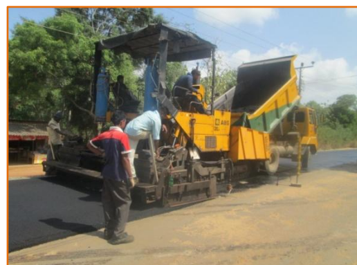
Asphalt concrete wearing course paving
