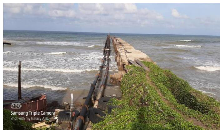
NEW SEA WATER LINE WAS LAID ALONG THE JETTY BY USING BLACK IRON PIPES
